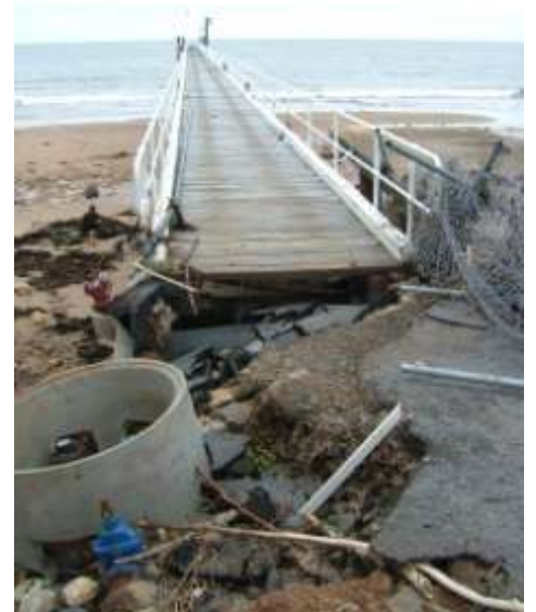
Above: Clump Point jetty after TC Larry in 2006 produced peak stillwater levels more than 2 m above the high tide levels between Cardwell and Cairns.
